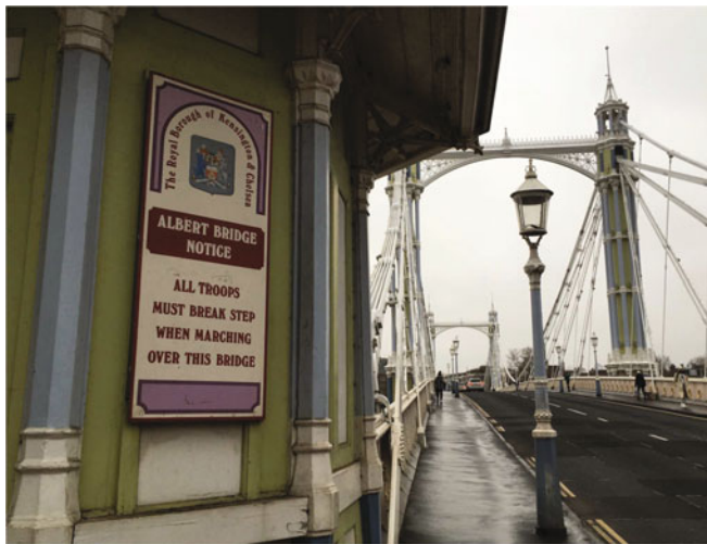
Figure 10.13. The Albert Bridge in London.
